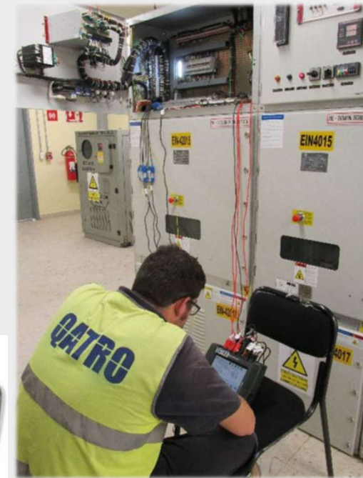
Technician conducting searches on a MV bar connection
